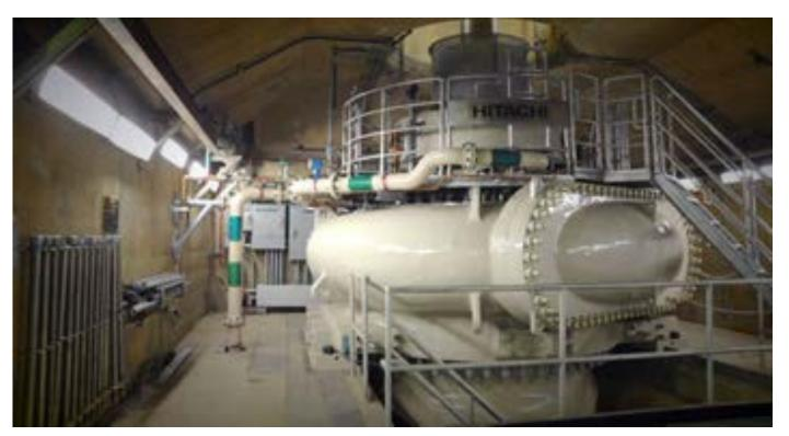
Vertical Multi Stage Centrifugal Turbine Pumps achieved the world's highest level of pumping efficiency while contributing to reductions in CO<sub>2</sub> emissions.
